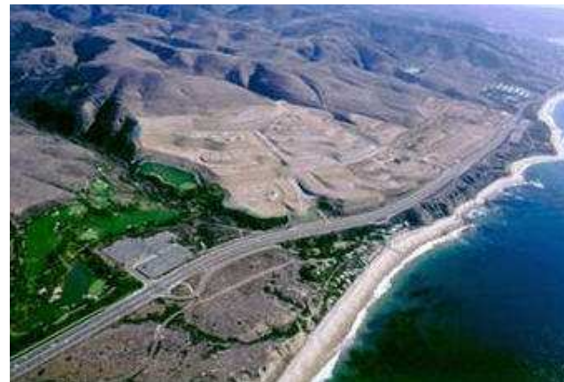
Rough Grading at Crystal Cove – Newport Beach, CA
