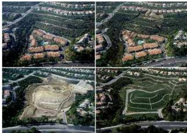
Laguna Niguel Side Slope Stabilization – Laguna Niguel, Ca.
